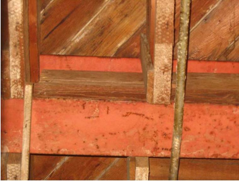
Figure 4. View from below of typical beam supporting second floor wood framing.
