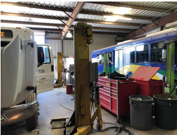
YCAT maintenance shop.
